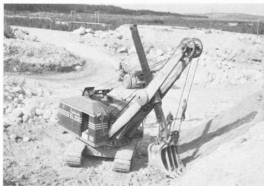
Fig. 2. Excavation of till with power shovel.
